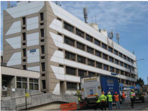
Police HQ building on the west side of John Street
